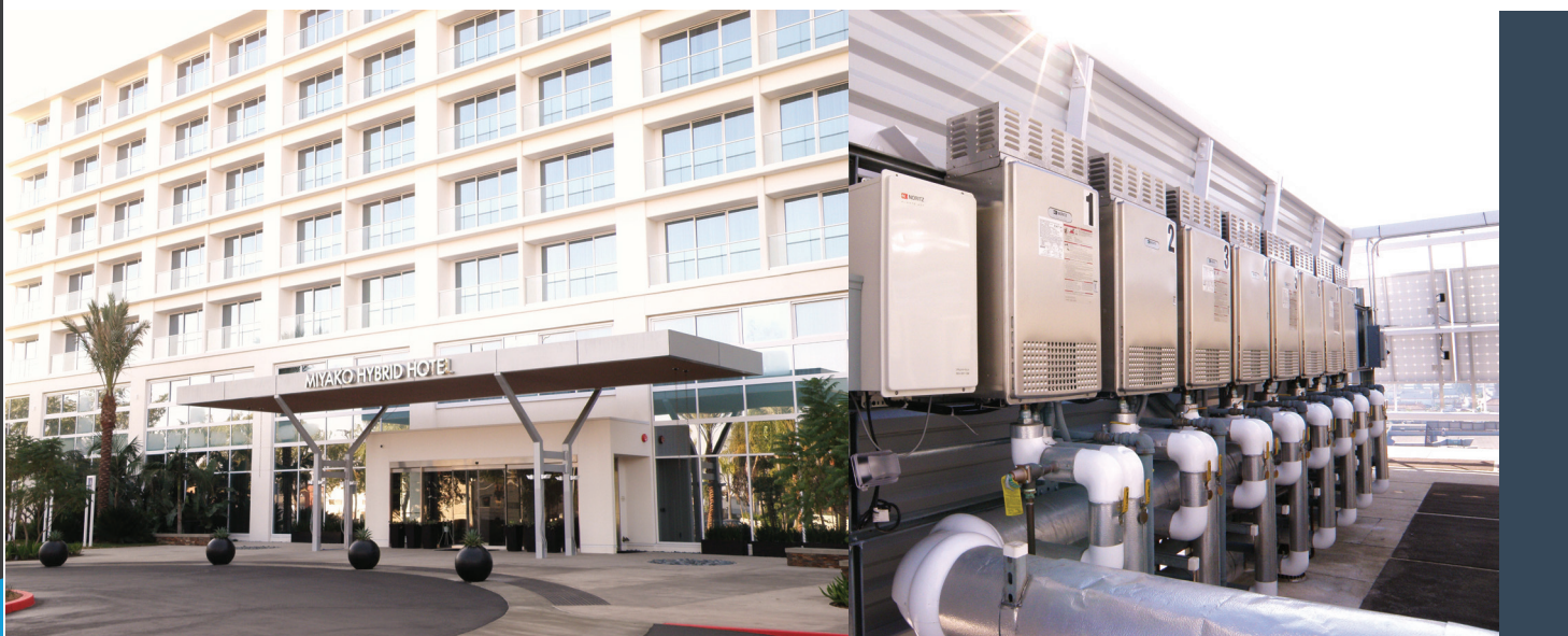
Miyko Hybrid Hotel Installation
